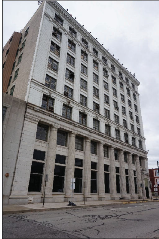
Photo 3. Subject building, The Peoples Bank, western elevation, facing east.
