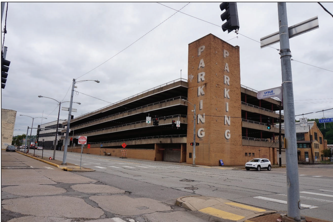
Photo 8. Lysle Boulevard Parking Garage, southeastern oblique, facing northwest.
