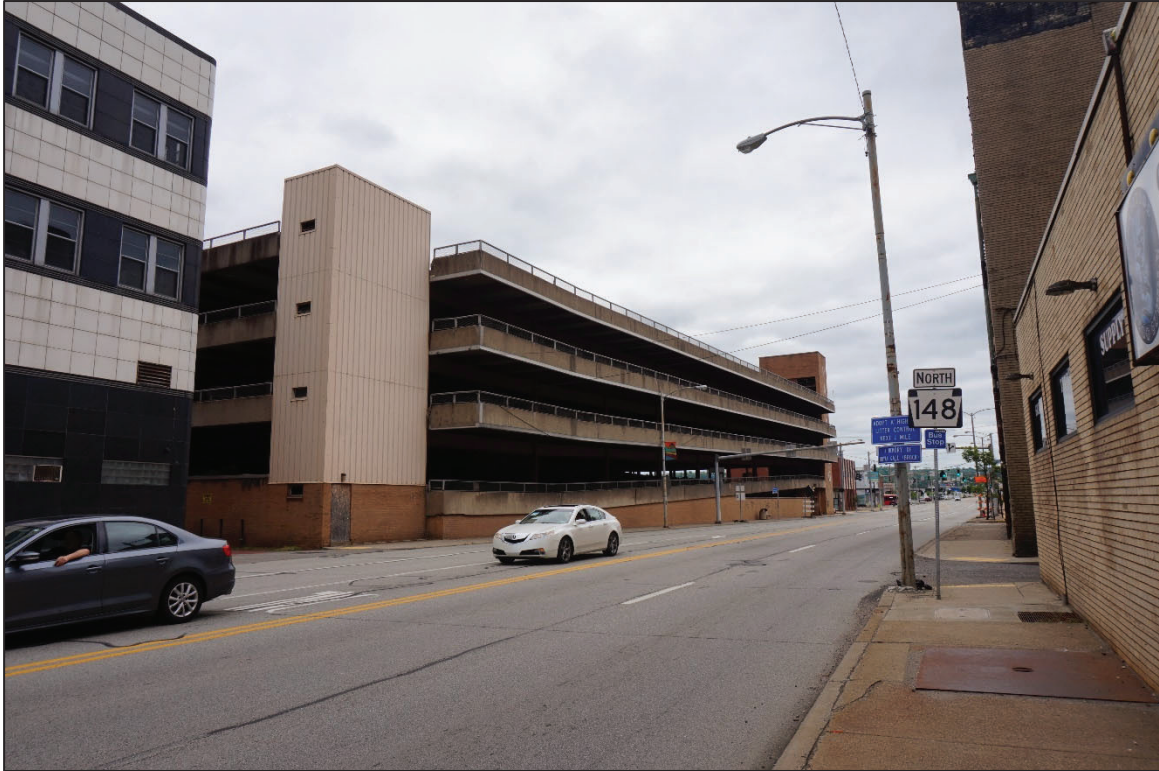
Photo 9. Lysle Boulevard Parking Garage, southern elevation, facing northeast.
