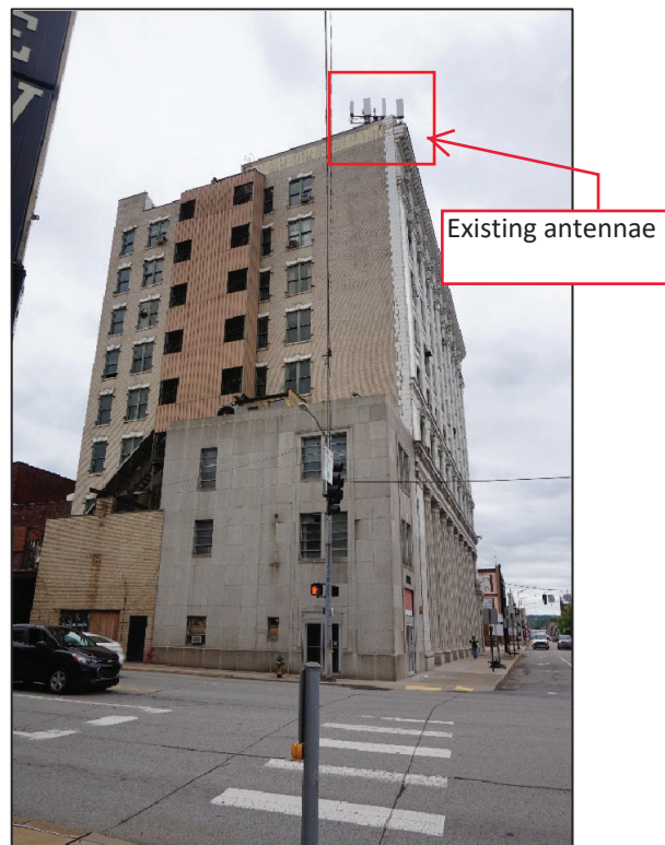
Photo 6. Subject building, The Peoples Bank, northern elevation, facing south.
