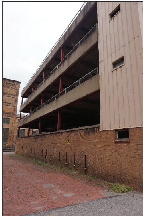
Photo 10. Lysle Boulevard Parking Garage, western oblique, northeast.
