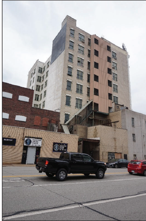
Photo 7. Subject building, The Peoples Bank, northeastern oblique, facing southeast.
