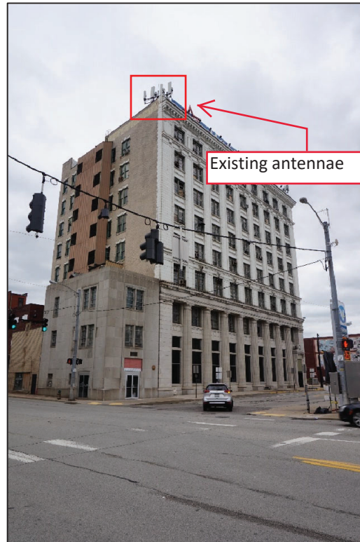
Photo 5. Subject building, The Peoples Bank, northwestern elevation, facing southeast.
