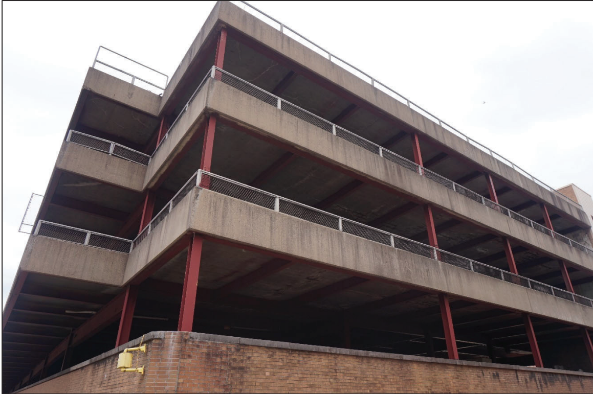
Photo 11. Lysle Boulevard Parking Garage, northwestern oblique, facing southeast.
