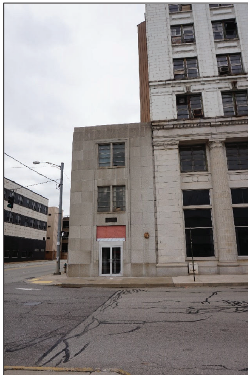
Photo 4. Rear commercial addition, The Peoples Bank, western elevation, facing east.
