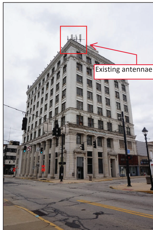
Photo 2. Subject building, The Peoples Bank, southwestern oblique, facing northeast.
